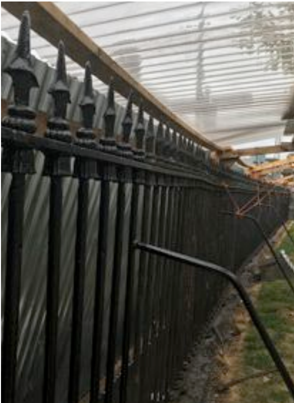
Temporary structure to protect from weather and for public safety, designed to move along as works progress
