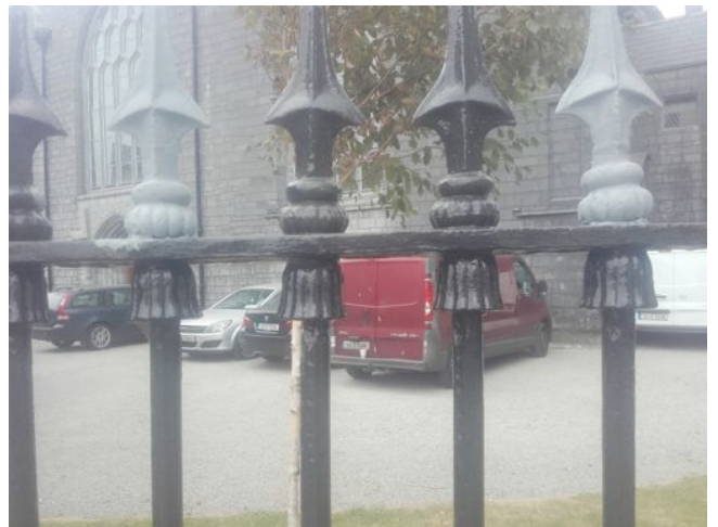
New finials cast and fitted prior to painting to both lengths of railings between south tower and Lynch's Window
