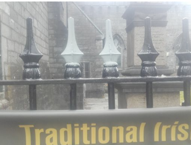
New finials cast and fitted prior to painting to both lengths of railings between south tower and Lynch's Window
